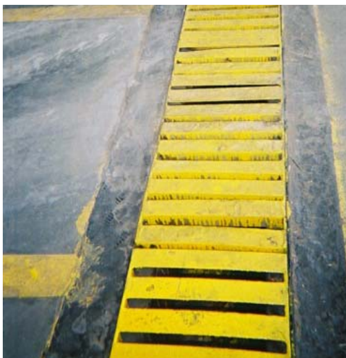
Pic. - Covered drainage channel at the Comercializadora de Baterias SA storage yard in the center of Mexico City.
