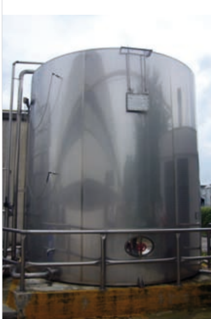
The project used a large balance tank to treat waste water
