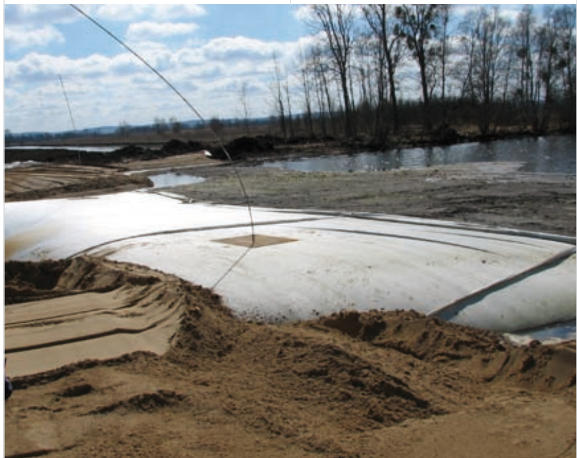
LIFE constructed a 7.3 km dyke that prevents water drainage
