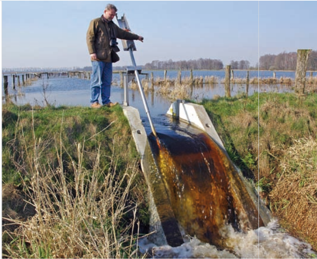
An adjustable weir enables better control of the water table
