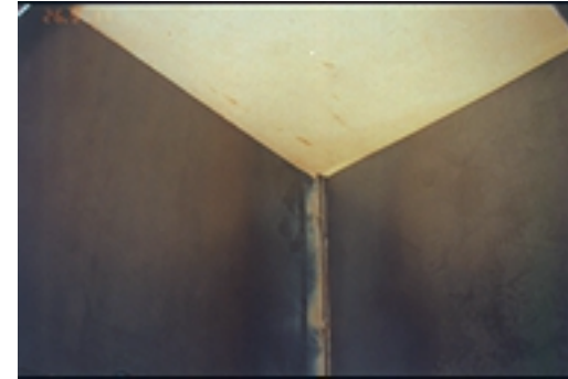
Photo : Welded Joints of Transit bins
