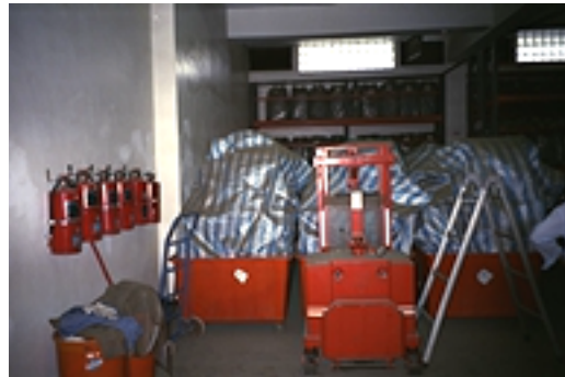
Photo : Fire Fighting Equipment
