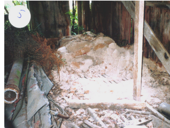
Photo: Old DDT store showing free form storage and leaking into environment
