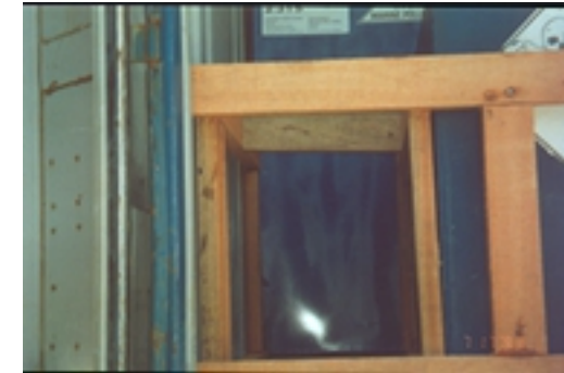
Photo : Container bracing, interior view
