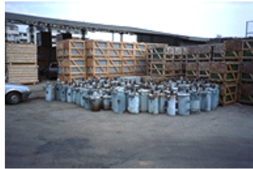
Photo : Hard Surface storage (PCBs) without environmental protection
