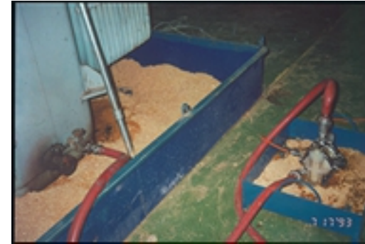
Photo : Temporary bunding for transformer decanting
