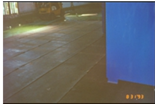
Photo : Floor Sealing in Containment area
