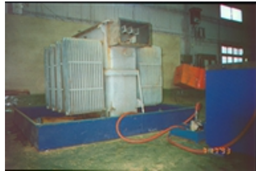
Photo : Decanting Power Transformer with temporary bund
